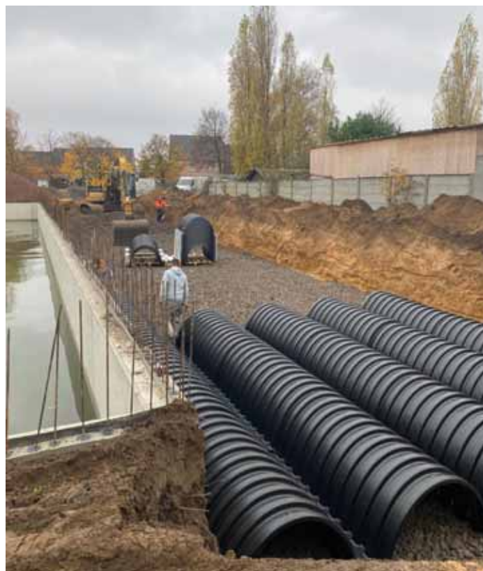
Postup instalace Pluvio PL1200
