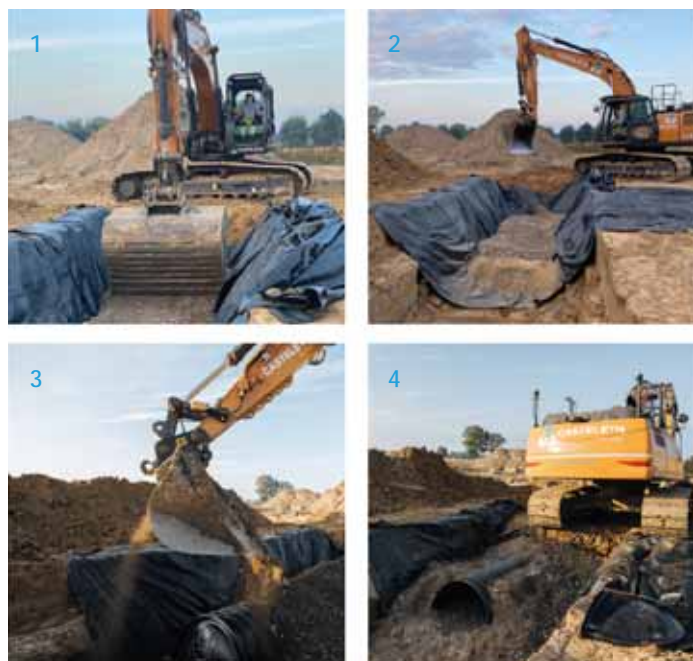
Postup instalace Pluvio PL1200
